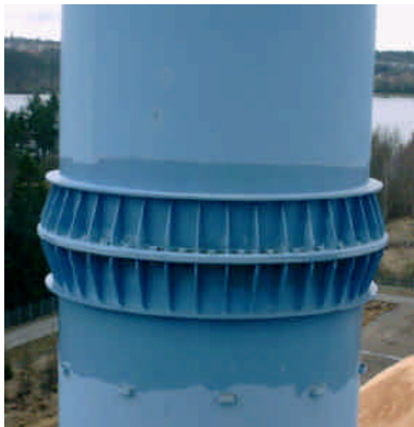
Figure 2.2 j The modified flanged erection splice at h=30 m level. Modification made in December 1998.
