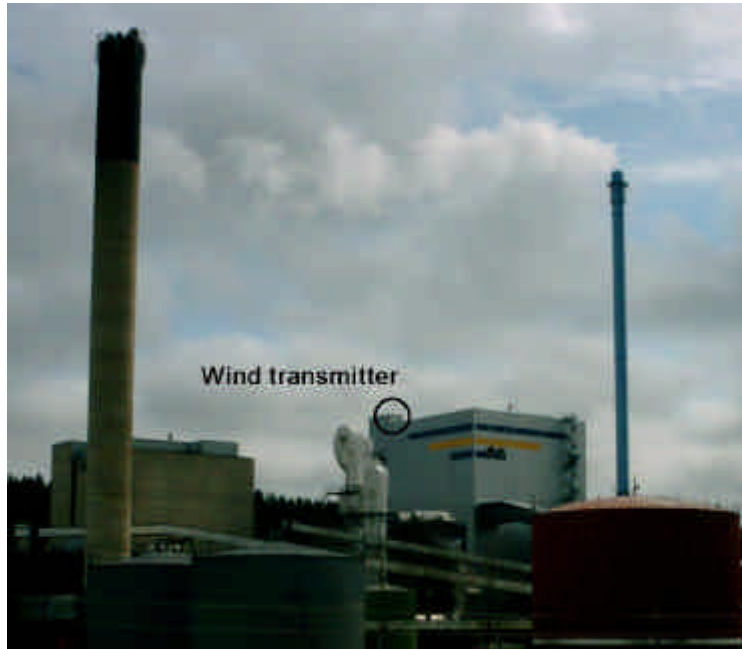
Figure 3.2 b The VEAB Sandvik plant. To the right Sandvik II unit and the 90 m steel chimney. A balloon shows location of the wind data transmitter on top of the power plant building of the Sandvik II unit.
