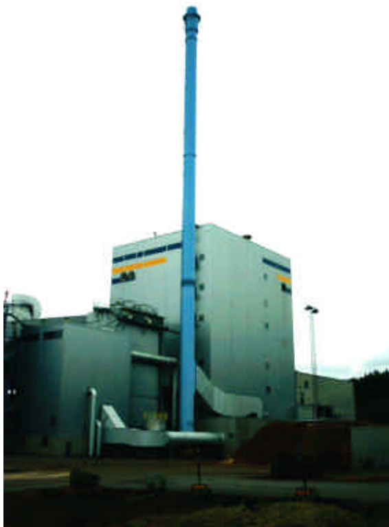
Figure 2.1 c The VEAB chimney from south showing neighbouring buildings.
