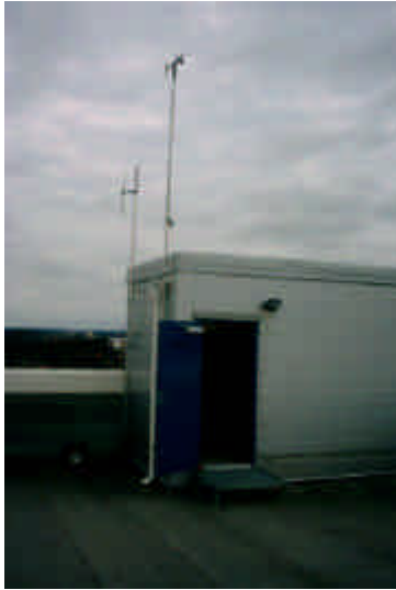
Figure 3.2 c The wind data transmitters on the Sandvik II unit roof.
