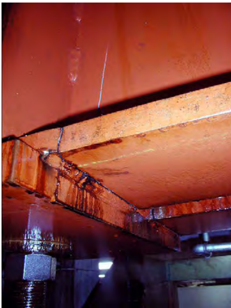
Figure 19. Fatigue cracks in two parallel hot-rolled beams HEB1000, initiated at the weld toe of the fillet weld to the cover plate at the lower flange and then propagating up to half the height of the web of the beams
