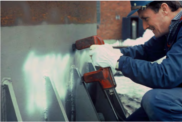
Figure 14. Magnetic-particle testing of welds at the base of the chimney in Figure 13. The lower part of the chimney made of weather-resistant steel has been blast-cleaned before testing
