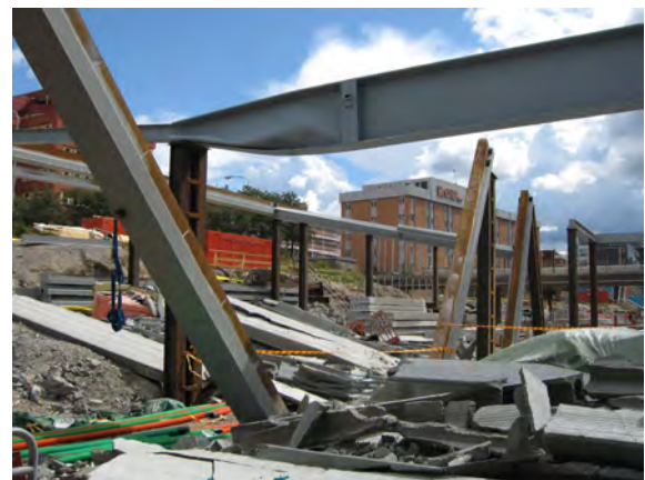
Figure 3. Welded 1400 mm high I-girder which initiated the structural collapse shown in Figure 2
