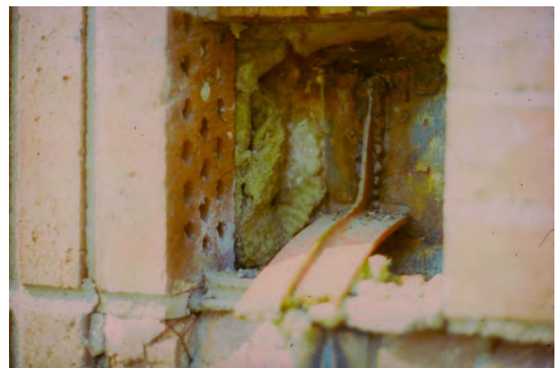
Figure 12. Detail of fractured welded attachment of cantilever beams for a roof over walkway
