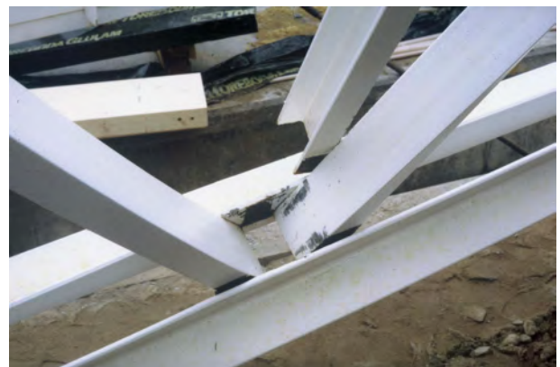
Figure 6. Joint in collapsed roof trusses from Figure 5, with some fractured welds
