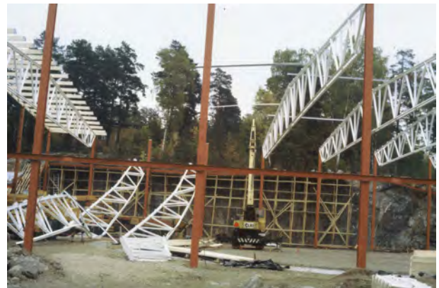
Figure 5. Roof trusses collapsed during construction when roof structure is being erected
