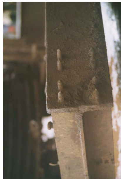
Figure 9. Detail of cross beam carrying the conveyor belt gallery in the process building, with bolts loaded in tension and damaged by corrosion
