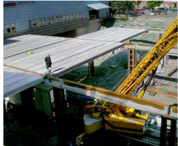
Figure 1. Commercial center building under construction, view half an hour before structural collapse
