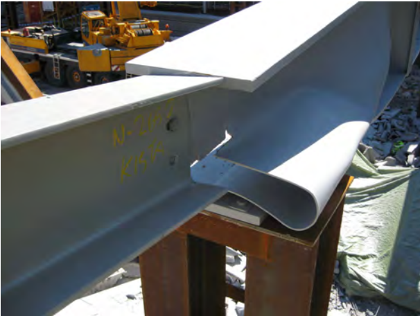
Figure 4. Local buckling of the web of the I-girder over the column support, where web stiffeners are lacking
