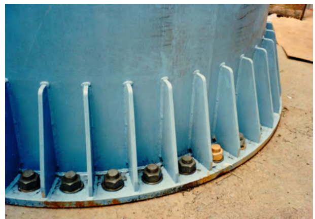
Figure 17. Base of 90 m high chimney with malfunctioning mass damper at the top
