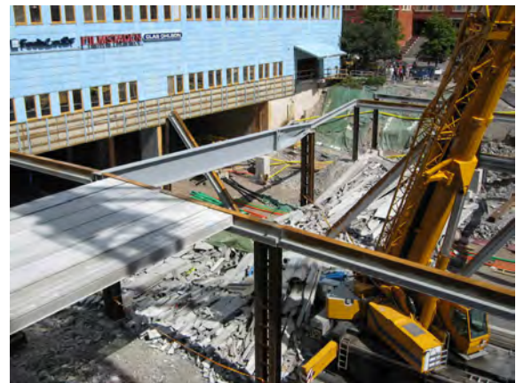
Figure 2. Same view as in Figure 1, after collapse
