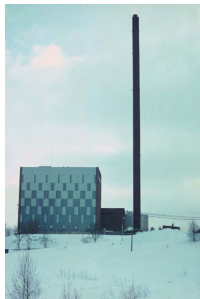
Figure 13. 90 steel chimney where fatigue cracks due to vortex shedding were detected at the base
