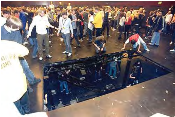
Figure 10. Collapsed floor deck in concert hall
