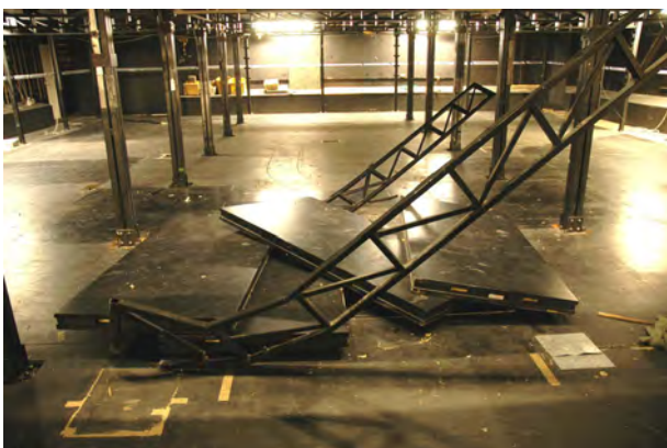
Figure 11. Collapsed steel truss beams in the floor deck of Figure 10
