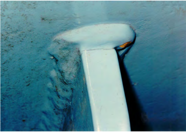
Figure 18. Example of fatigue crack at a stiffener at base of chimney shown in Figure 17, in this case visible in the cracked paint
