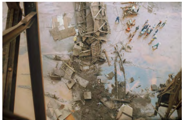
Figure 8. Remains from collapsed conveyor belt gallery seen from a 30 m level in process building
