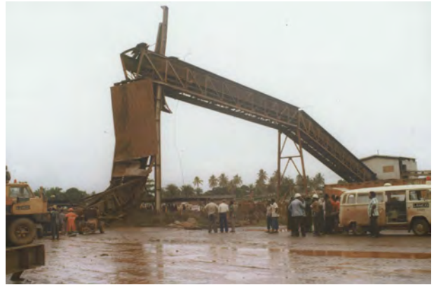
Figure 7. Collapsed conveyor belt gallery
