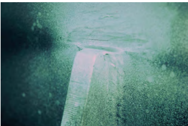
Figure 16. Fatigue crack indicated by magnetic-particle testing after grinding the detail in Figure 15 down to half the thickness of the shell plate
